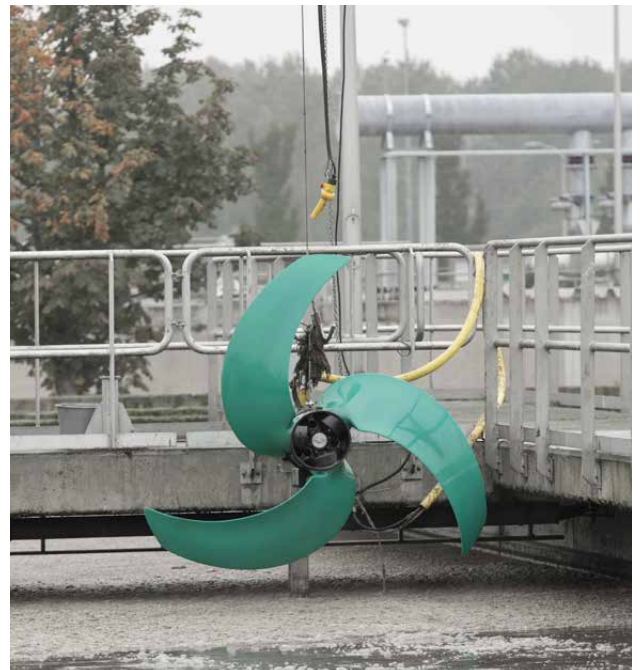
Lowering devices for optimum positioning in the basin
