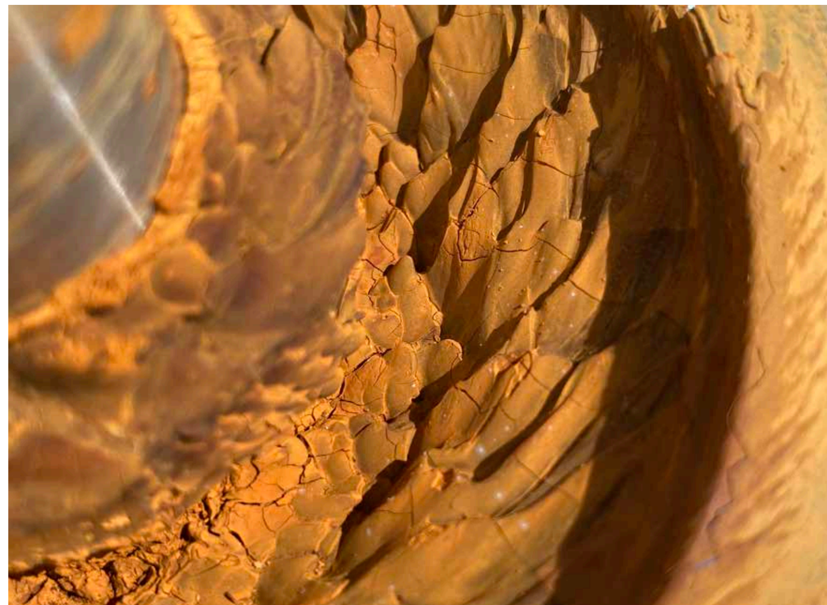
Pump with heavy iron oxide deposits
