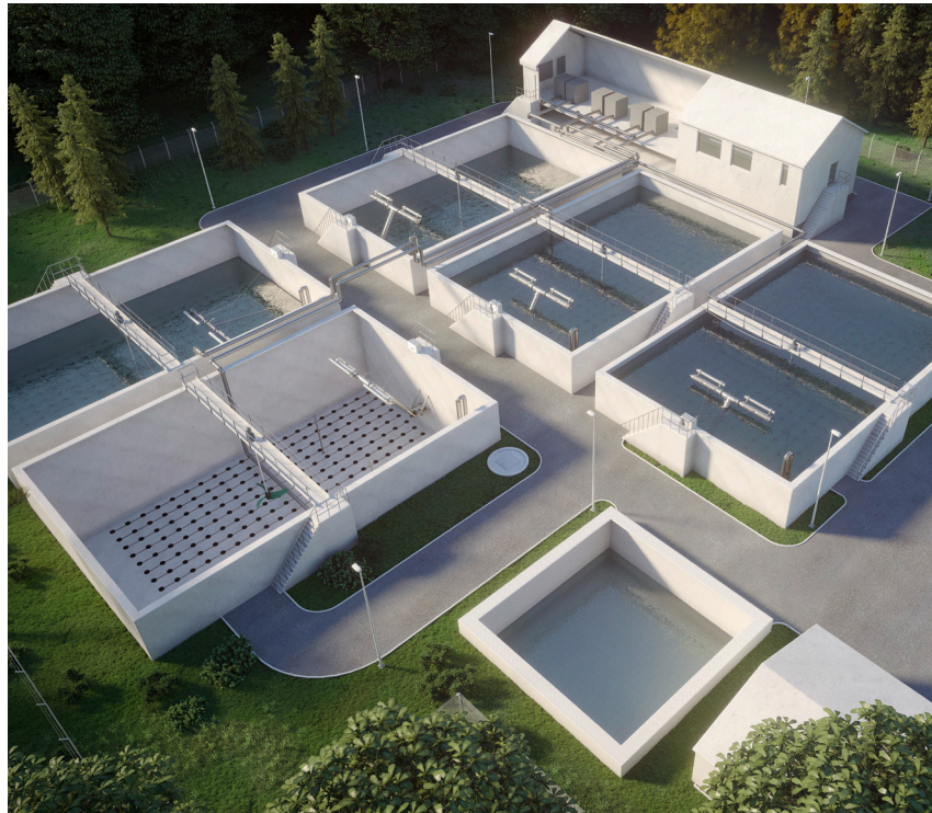
The SBR process at a glance. In every SBR reactor, conversion of the sewage constituents and sedimentation of the activated sludge required for this process takes place in a cyclical sequence.
