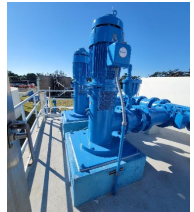
Figure 1: American Marsh Vertical Turbine 14MFLZ-1 Back Wash Pump
