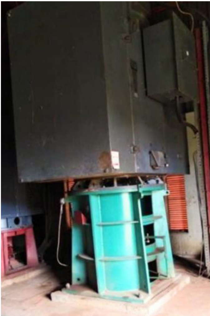
Caption: Rehabilitating Akute Water Intake in Lagos, Nigeria – Installing next-generation Wilo Vertical Turbine Pumps to enhance water supply efficiency and resilience
