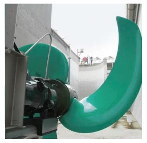
A **submersible mixer** is a machine designed to operate fully underwater in tanks, basins, and other liquid volumes to keep liquids and solids in motion. By creating circulation, it ensures even mixing, prevents sedimentation, and supports biological and chemical processes. Submersible mixers are widely used in sewage treatment plants, sludge tanks, equalization basins, and industrial applications, where they provide reliable mixing for agitating, blending, dissolving, and suspending solids.
