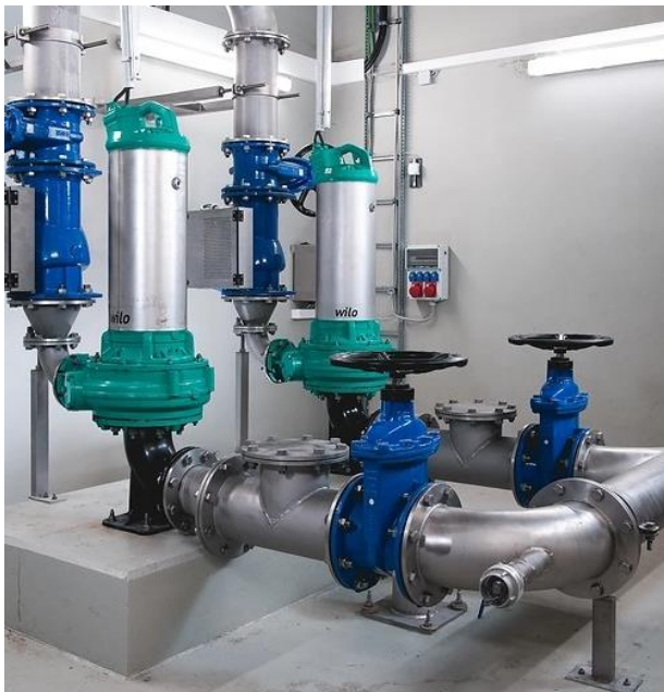
Wilo-Rexa SOLID submersible pumps in an enclosed dry-pit installation
