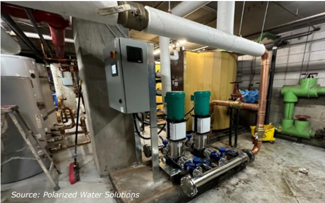
Newly installed Wilo-CO 2 Helix at Barclay Towers
