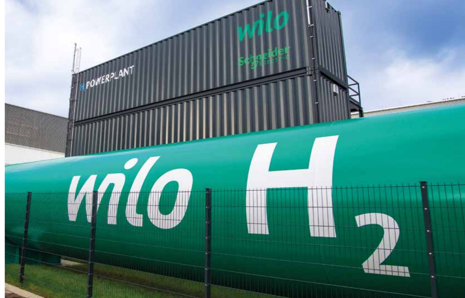
The H 2 POWERPLANT pilot hydrogen facility at the Wilopark, the company's headquarters in Dortmund, is an important element of the Wilopark energy concept, as it stores the electricity generated by the photovoltaic system on the factory roof and then distributes it when it is needed.
