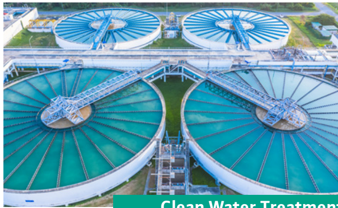
Clean Water Treatment
