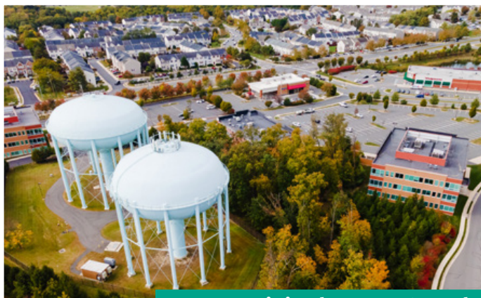
Municipal Water Supply
