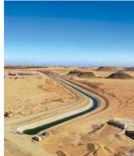
In the Egyptian Toshka project, Wilo products and systems are helping to turn desert into land for agricultural purposes.
