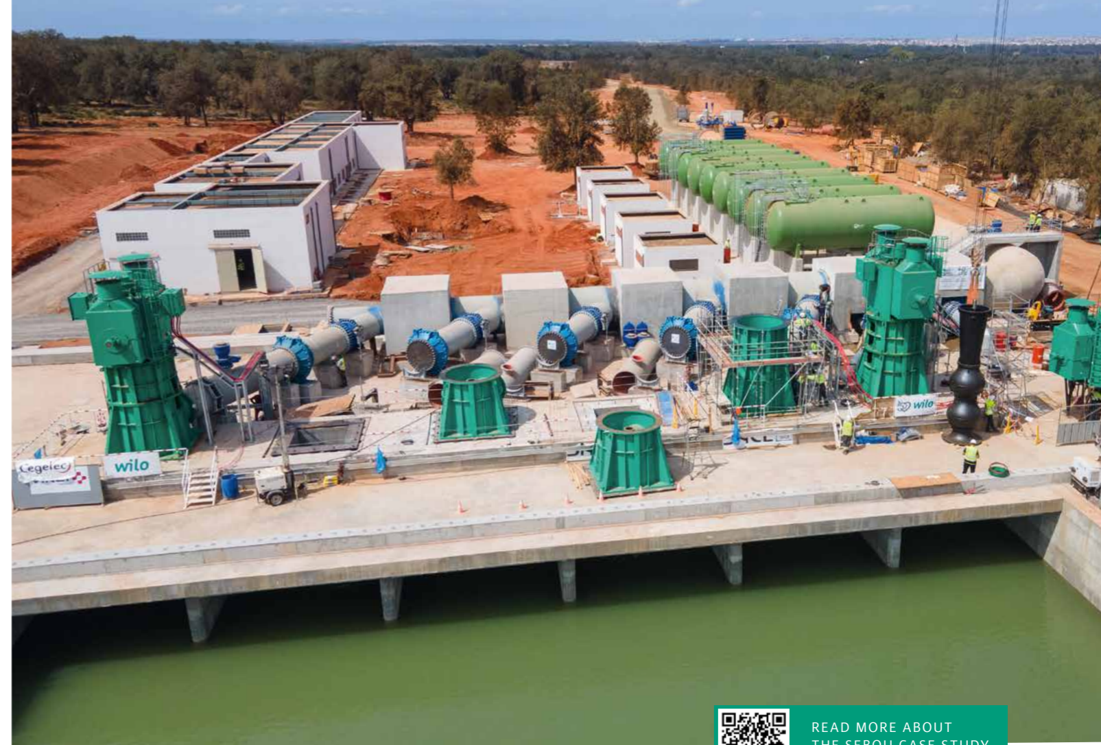
Twelve vertical turbine pumps connect the Sebou dam to the Sidi Mohamed Ben Abdellah dam to secure the drinking water supply for the major cities of Rabat and Casablanca.
