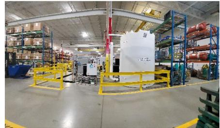
Figure 2: Wilo USA Rainwater Collection Tank & QuantumFlo Booster Pump
