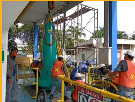
Installed Pump : – Water Distribution Pump
