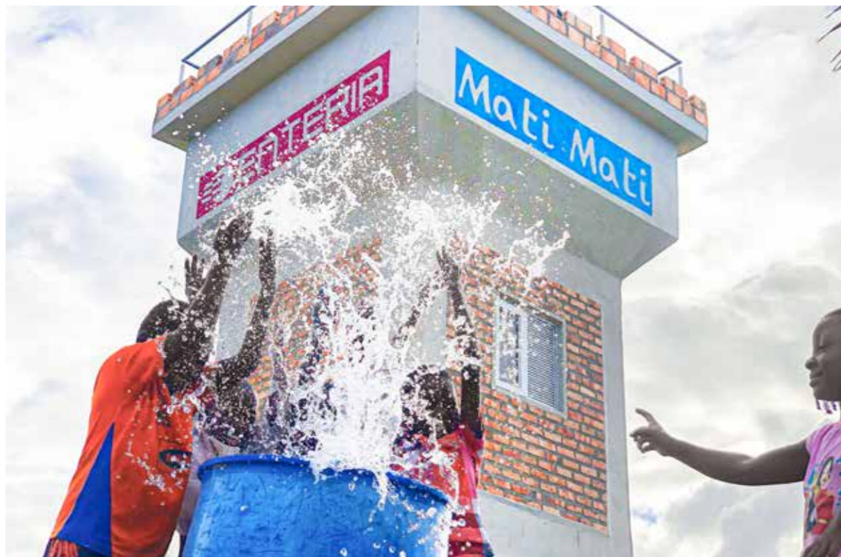
Water tower in Pebane, Mozambique
