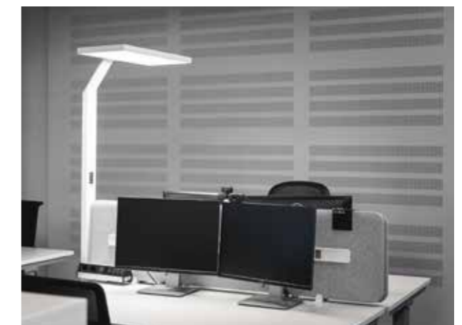
The lighting in the new offices at the Dortmund site also measures air quality
