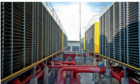
Chillers, cooling towers
