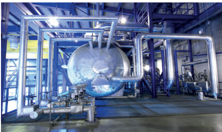
Hot water, steam boilers and CHP
