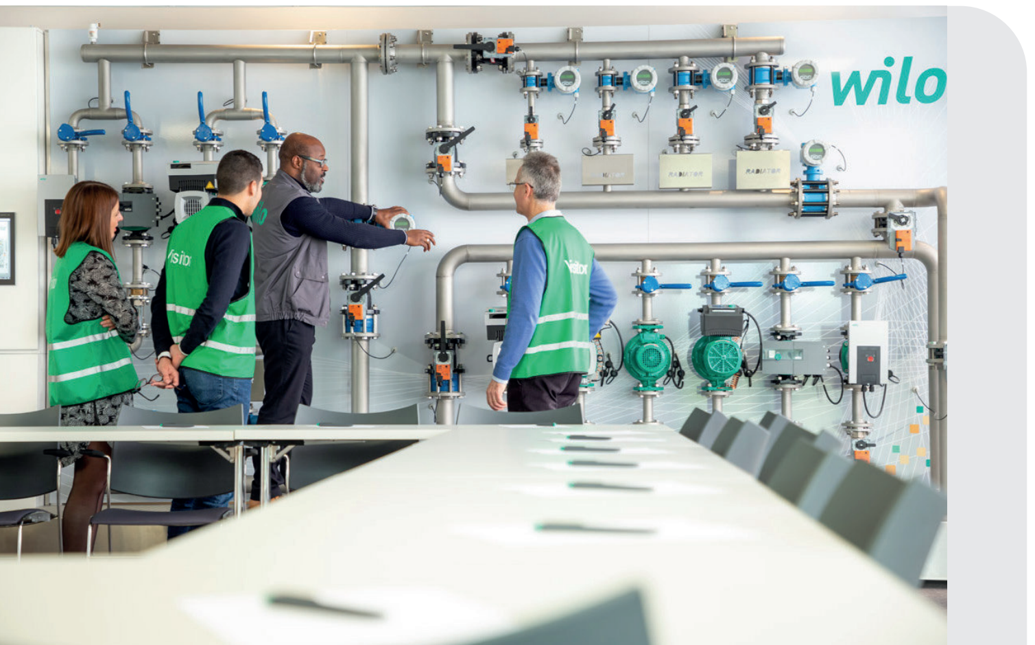
Training loop installed in Aubigny (France)
