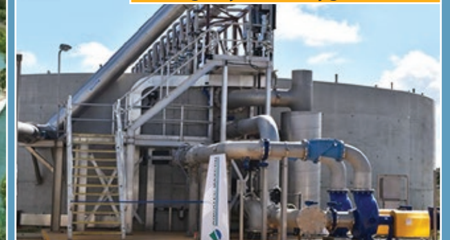
Kingaroy WWTP Upgrade AUS
