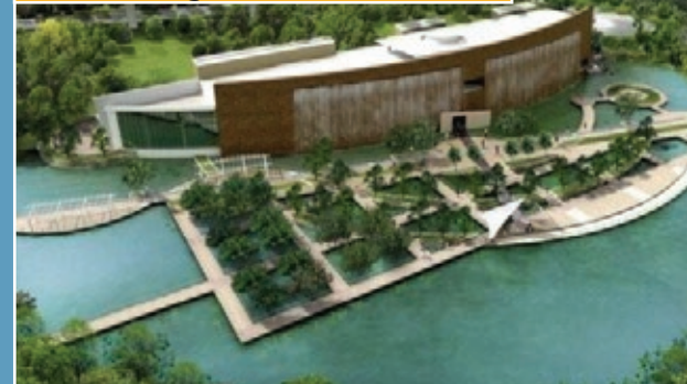
WWTP Bangsu – Thailand
