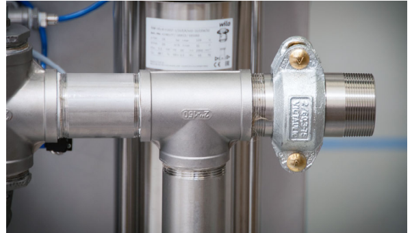
Process water pipe connection
