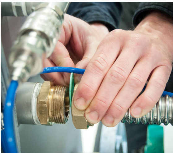
Connection of overflow line to tank.
