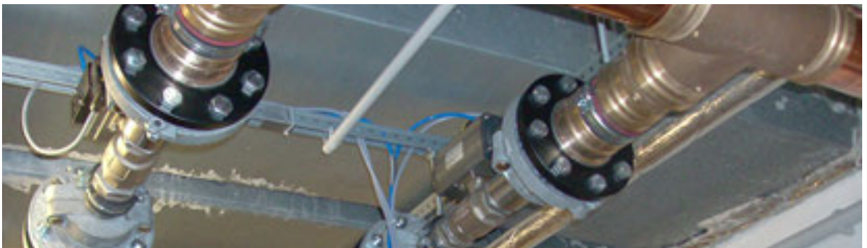
Exemplary connection of pump emergency drainage to drainage installation.
