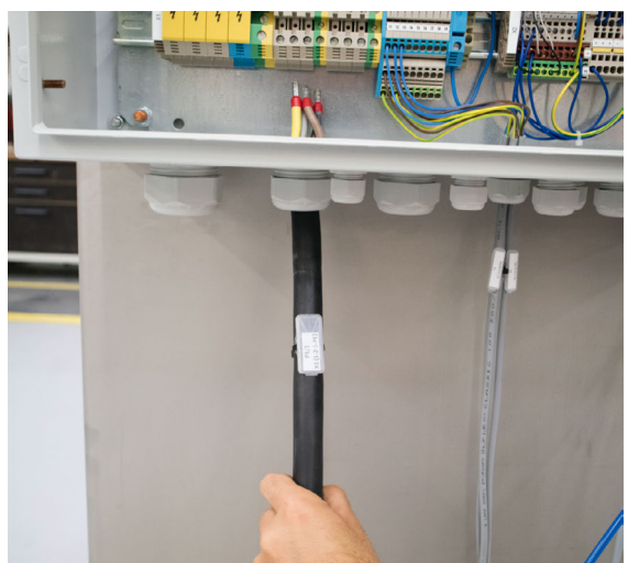
Guide the cable into the control unit.
