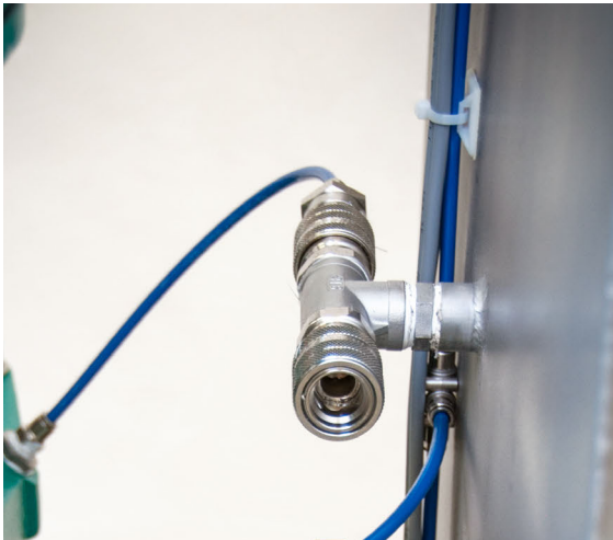
Connection of pump vents to quick-release couplings tank.
