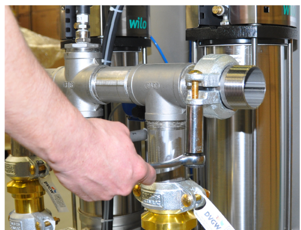
4. Connect and tighten the coupling. The grooves of the coupling grip into the roll groove seam.
