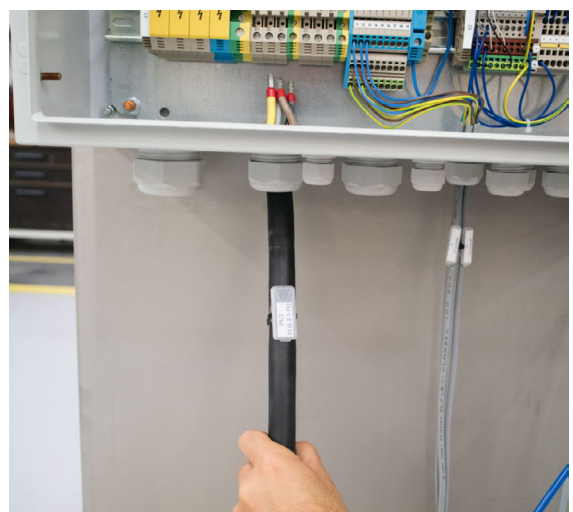
Guide the cable into the control unit.
