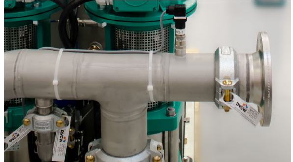
Process water pipe connection
