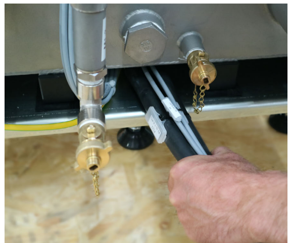
Guide the cable harness centrally under the tank.
