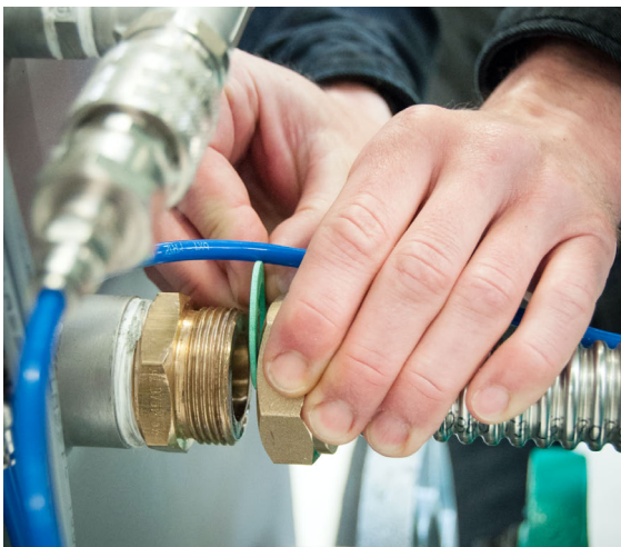
Connection of overflow line to tank.
