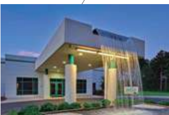
WILO USA LLC Thomasville, Georgia, USA
