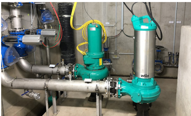
Thanks to the use of Wilo-Rexa SOLID-Q with Nexos Intelligence when modernising the pumping station Buchbusch, cloggings could be greatly reduced thus service calls have also been minimised. Operating costs could be significantly reduced.
