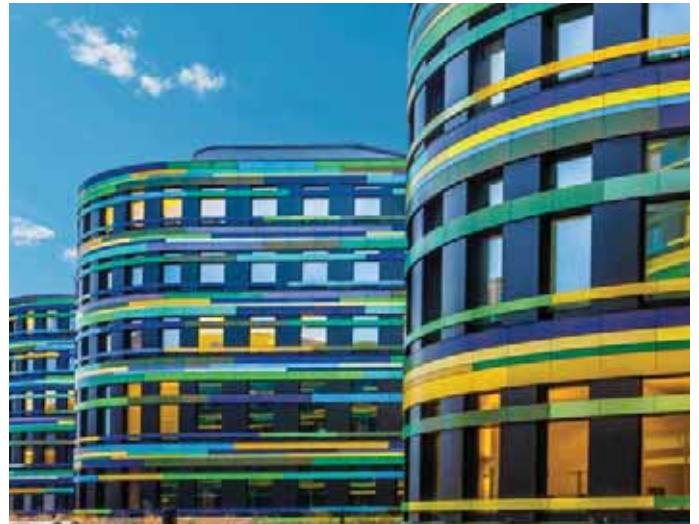
Building of the state ministry for urban development and the environment - Hamburg - Germany
